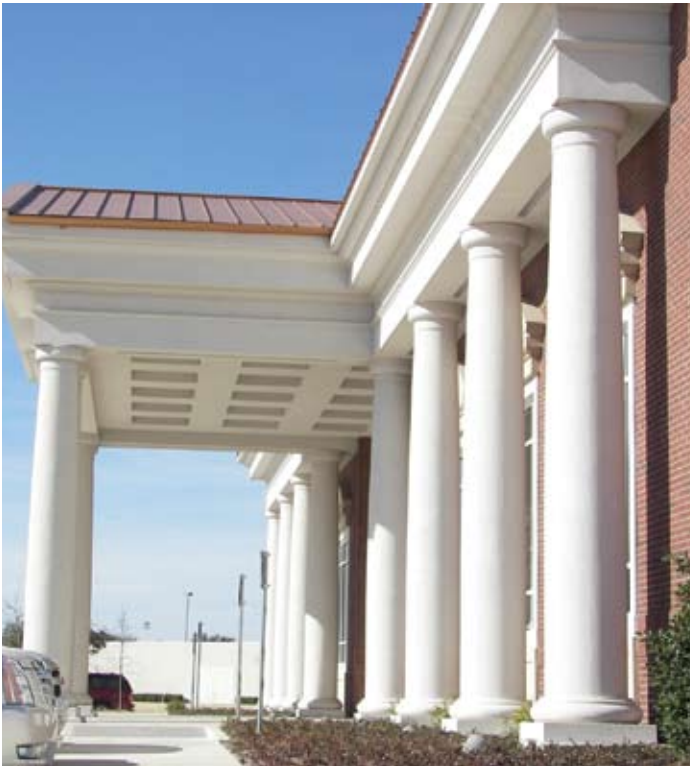
▲ Exterior Round Stacking Columns
